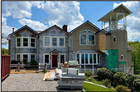
Rednal in the midst of the exterior renovations.
